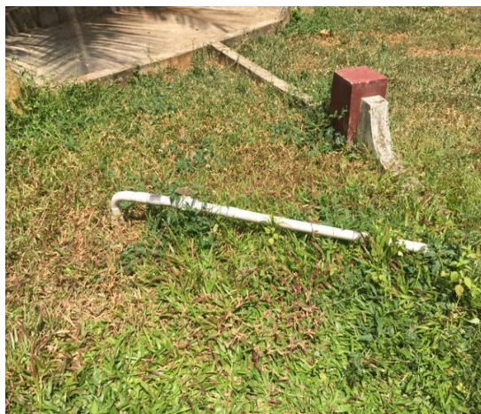
Figure 2: Bio gas plant
